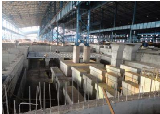
Plate Mill - Latest Site Pictures
