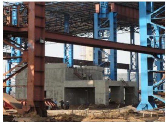
Steel Melting Shop - Latest Site Pictures
