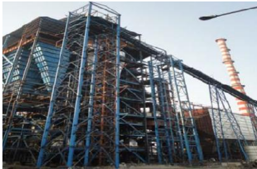
Power Plant - Latest Site Pictures
