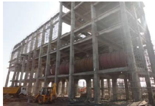
Sinter Plant - Latest Site Pictures
