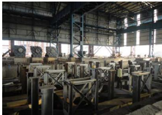
Rebar Mill - Latest Site Pictures
