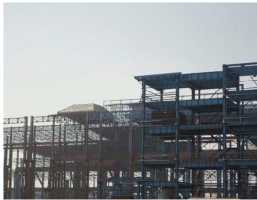
Steel Melting Shop - Latest Site Pictures
