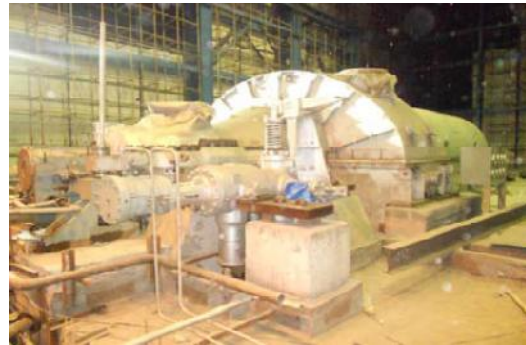
Power Plant - Latest Site Pictures
