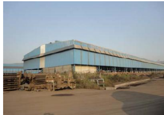
Plate Mill - Latest Site Pictures
