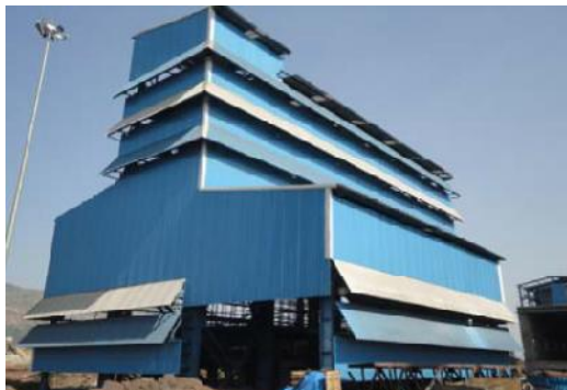
Sinter Plant - Latest Site Pictures
