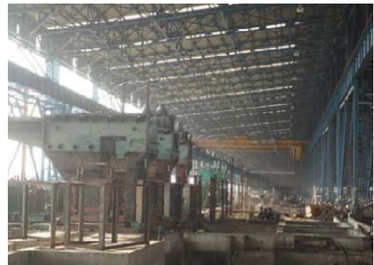
Rebar Mill - Latest Site Pictures
